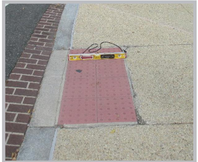
A curb ramp is measured with a slope meter.
