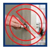
• DON'T tape over latches. During a fire, hot gases can easily build up enough pressure to blow fire doors open, rendering them ineffective.
