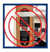
• DON'T cover door labels. A fire door and frame can often be identified by a labeled plate, indicating the laboratory approval and the duration of fire rating. Painters and maintenance crews should avoid covering or tampering with these plates.
