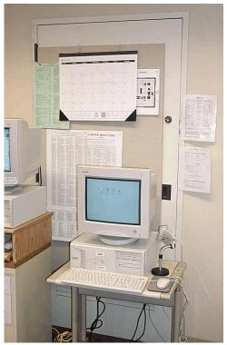
To the left is an electrical closet in a Congressional facility. The door is blocked by computers and office furniture. An added hazard is the lack of clear signage for the closet or any designation as to whether the panels inside are up to date or in serviceable order.
