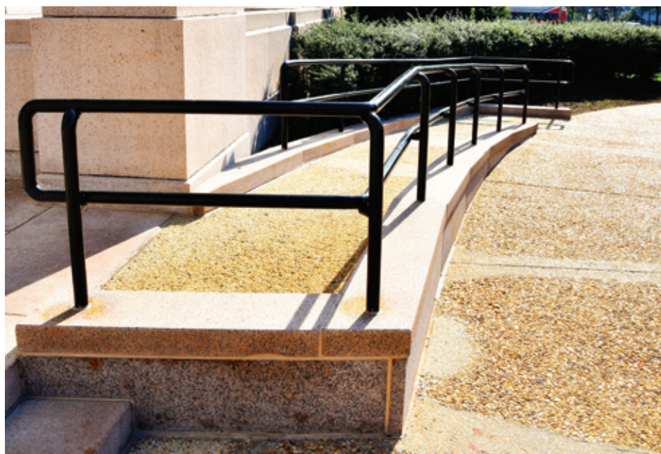
ADA inspections conducted by the OOC include reviewing exterior pathways.
