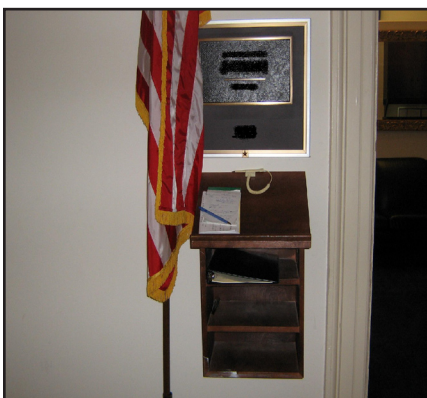
Figure 3: Braille signage not approachable within three inches
