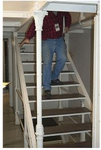
To the left is a stair that does not have a handrail where required. The man walking down the stairs is reaching for a handrail that is not there. He could easily tumble down the stairs and seriously injure himself if he lost his balance.
