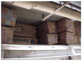
To the left is an example of an unacceptable practice with sprinklers. Creating an opening in the storage around a sprinkler does not satisfy code requirements because the sprinkler water is still blocked from reaching the wall.
