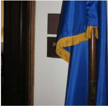
Image 3: Flag placed in hallway is blocking access to the tactile room sign.
