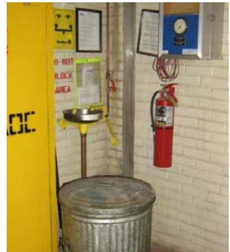
Figure 2: Obstructed Access to an Eye Wash
