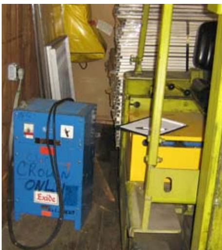
Figure 1: Battery Charging Station for a Forklift with Blocked Non-plumbed Eye Wash with Inspection Tag Attached
